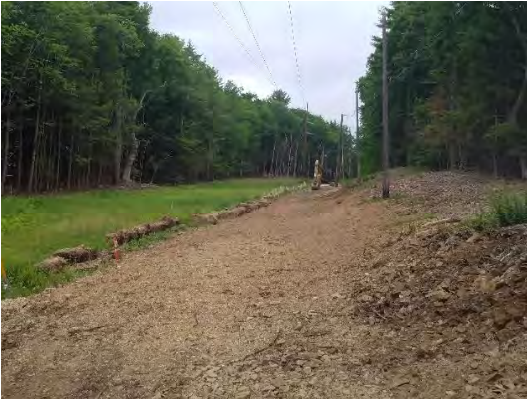
Fig 1: Removing gravel access road between Strs. 97-98. Viewing northwest. (06-25-20).
