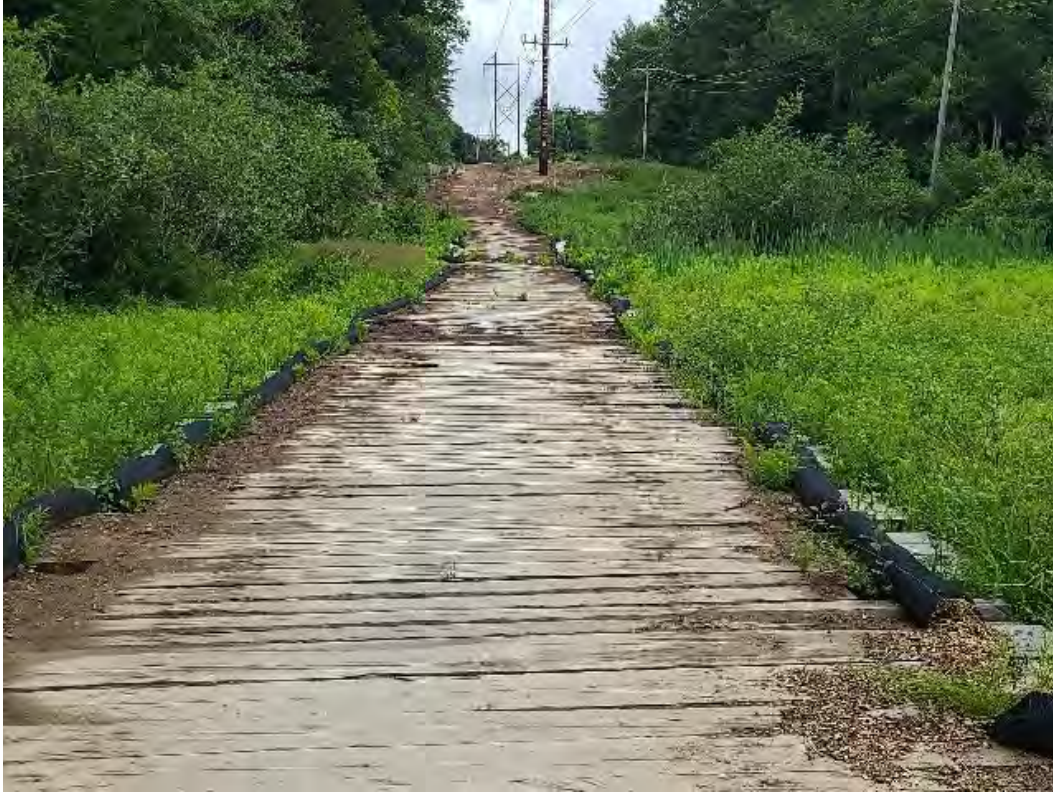
Fig 11: Access road through wetland DW33. Viewing northeast. (06-30-20).
