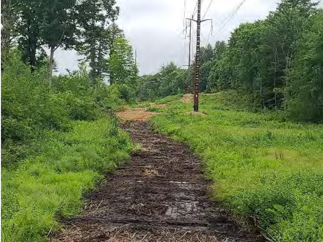
Fig 9: Crew removed timber mats from Wetland DW45, between Strs 39 and 40. Viewing north. (06-30-20).
