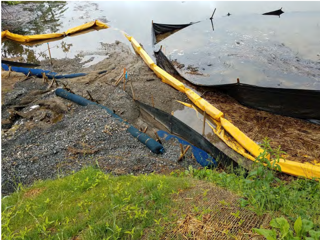
Fig 14: Gravel path erosion and deposition into the intertidal zone at Gundalow landing/east side of the Bay. Viewing southwest. (07-01-20).
