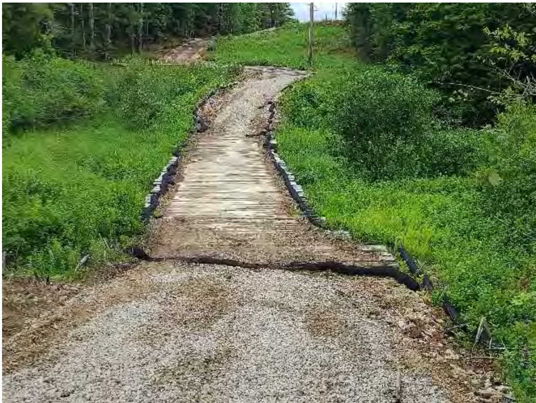
Fig 10: Access road over stream DS46, between Strs. 51-52. Viewing northeast. (06-30-20).
