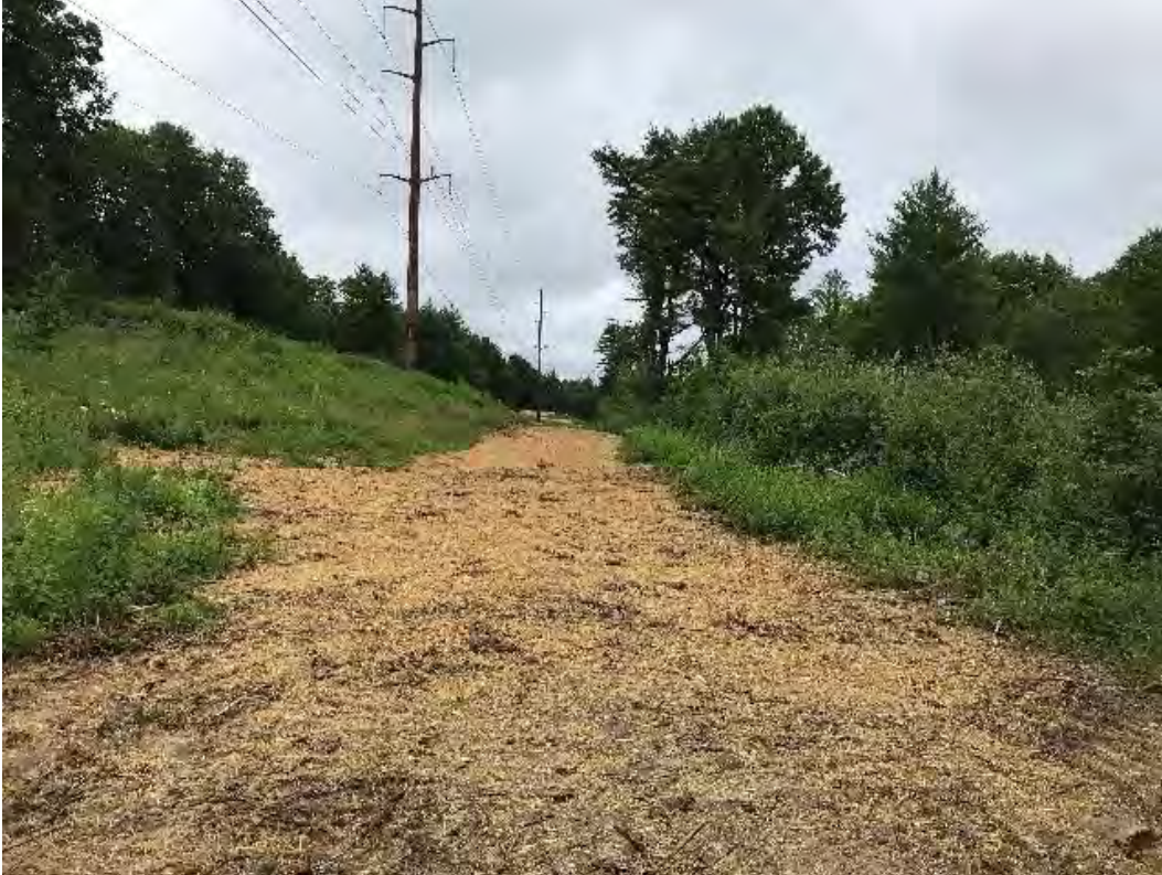
Fig 7: Restored access road between Strs. 44-43. Viewing north. (06-29-20).
